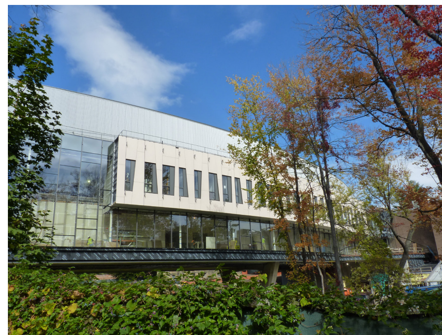
Above | Vassar College, Integrated Science Commons, Poughkeepsie, New York. Designed by Ennead Architects. © Arnold Glas
